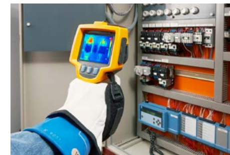
Predictive Maintenance (PdM) is giving manufacturers a more efficient, data-driven method for managing routine equipment maintenance.
